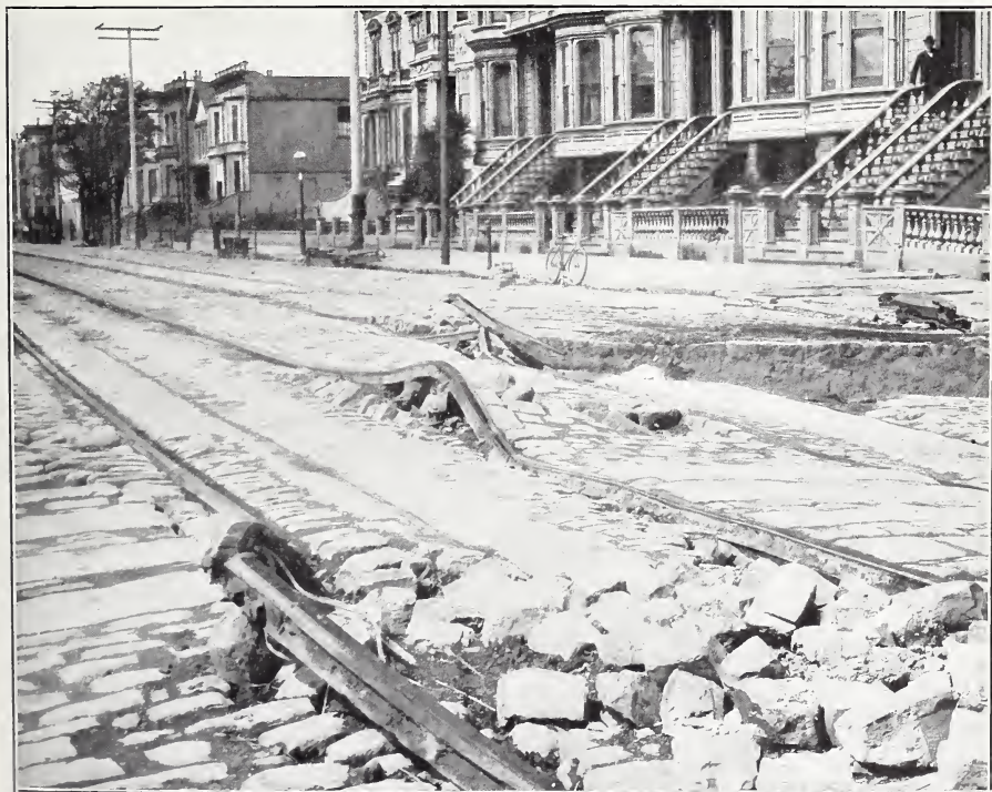
B. BUCKLING CAUSED BY EARTH FLOW, HOWARD STREET, SAN FRANCISCO.
